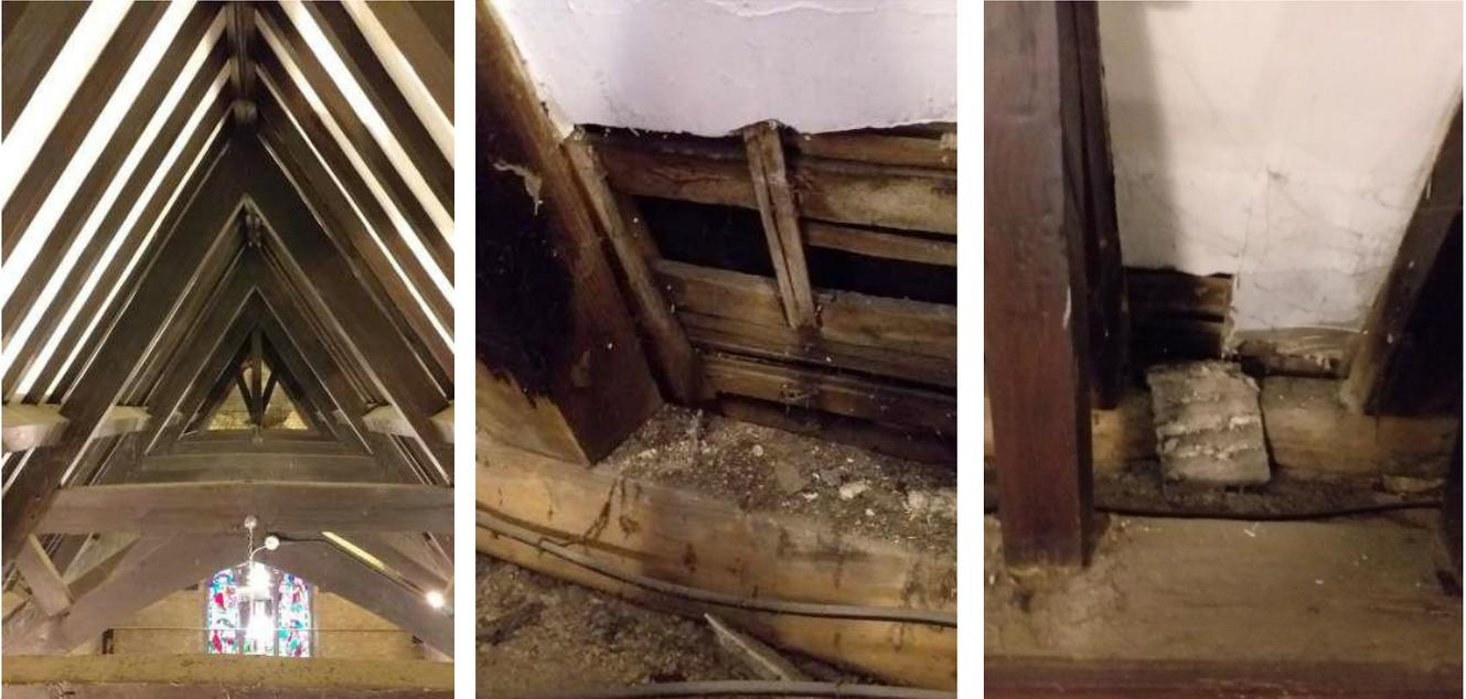
The nave ceiling was also inspected and it was found that all the panels had modern plasterboard fixed between the rafters and therefore was therefore it was considered to be sound requiring no further investigation.
